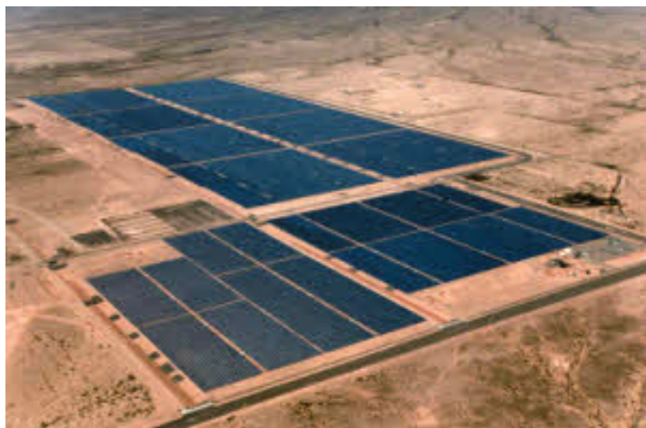
Soaring solar: An aerial view of Mesquite Solar 1 near Phoenix, Ariz., which powers nearly 56,000 homes.
