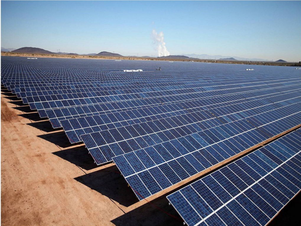
Capturing solar energy: Sempra U.S. Gas & Power has completed construction of Mesquite Solar 1, the first 150-megawatt (MW) phase of the company's Mesquite Solar complex, located near Phoenix, Ariz.
